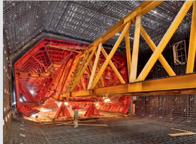
Internal formwork moves hydraulically over the launching beam.
