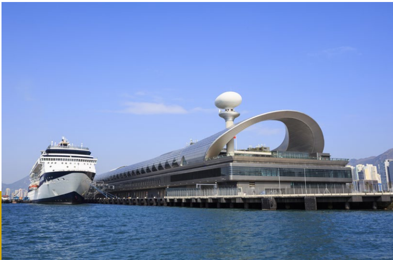
Kai Tak Cruise Terminal Building - Client: Dragages Hong Kong Architect: Fosters and Partners (Image courtesy of ROF Media)
