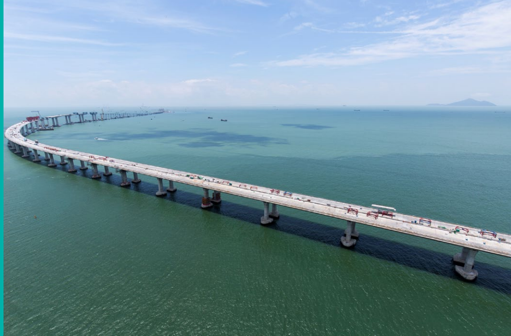
Boundary Crossing Facility, HKSAR
